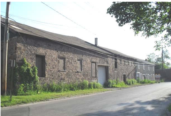
View of site looking east
